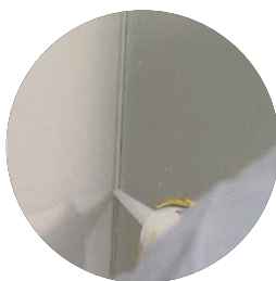
Note: Run Silicone down internal corner for water proofing.
